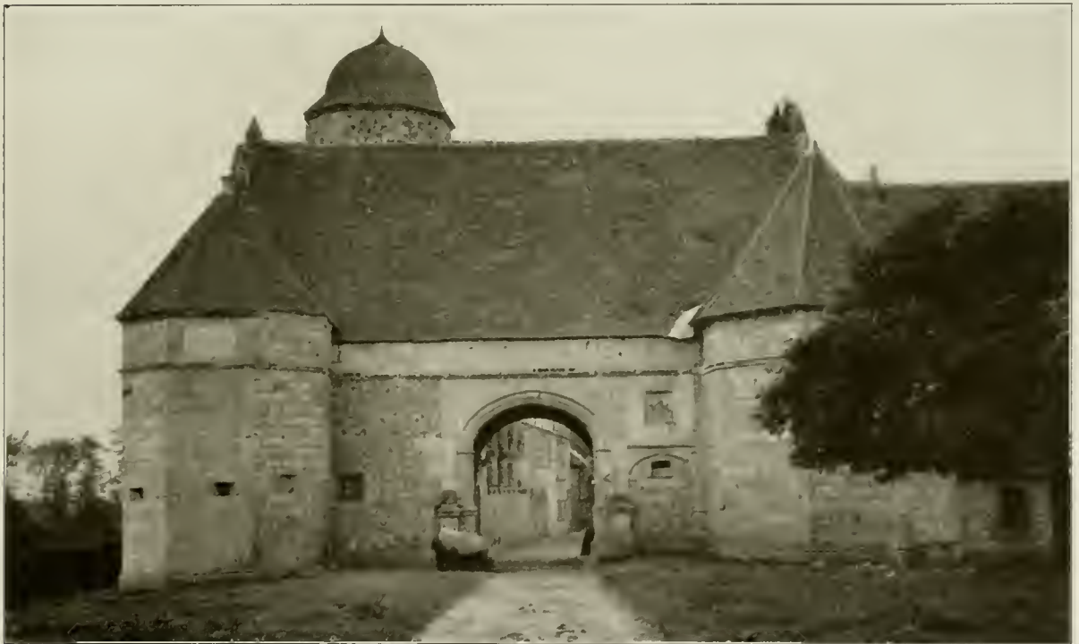
PLATE 104. Entrance to courtyard, Manoir d'Ango, Varengeville, Seine-Inférieure
